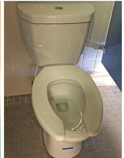
Shower heads and toilets were updated with more efficient EPA WaterSense labeled devices.
